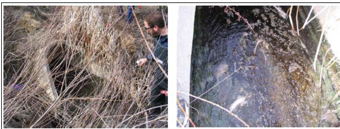
Photos 1 and 2. A dry weather sanitary survey resulted in identification of an illicit discharge to the storm sewer due to a plumbing error at a residential home. Toilet paper, odor, elevated temperature and other factors lead to identification and removal of this discharge.
