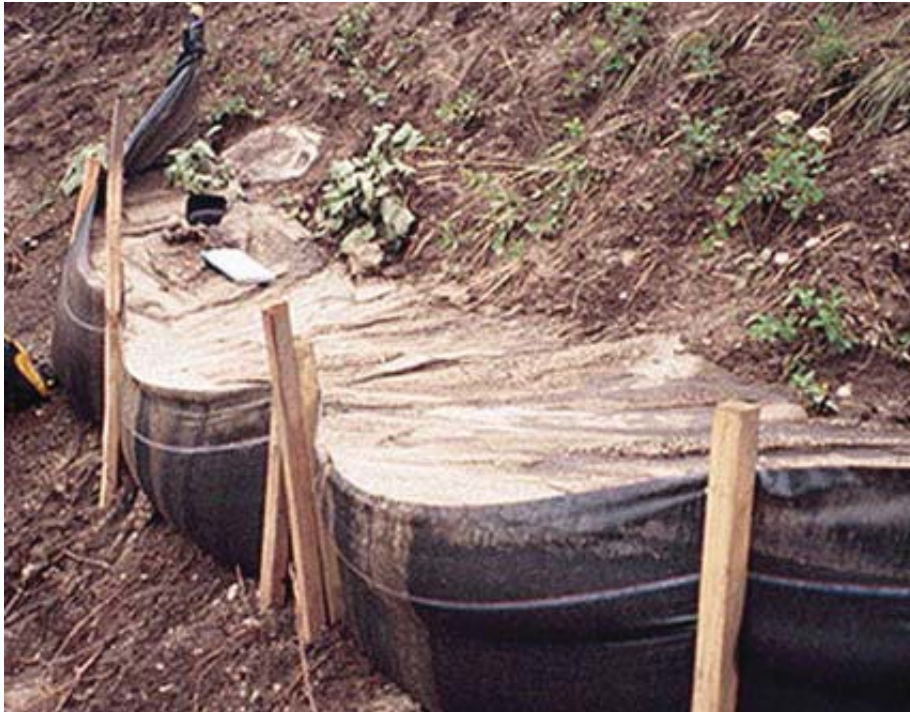
Figure B-6 Fully loaded silt fence placed after the 2000 Bitterroot Valley complex wildfire
