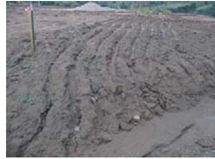
Grooving up and down the slope facilitating erosion
