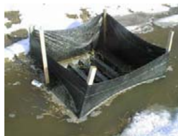
Drop Inlet protection made from silt fence
